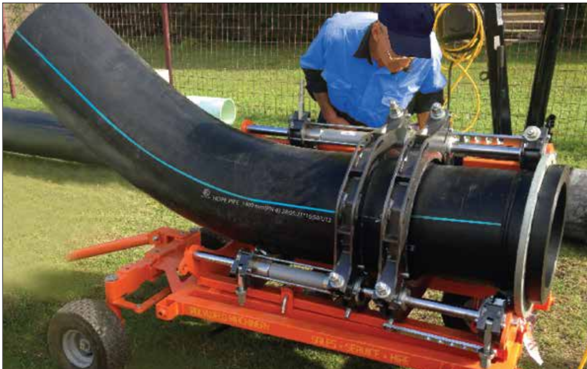
Butt Fusion Welding
