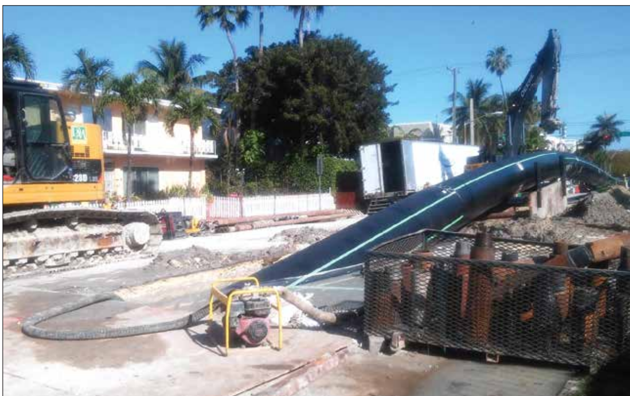
RFL HDPE Pipe Laying
